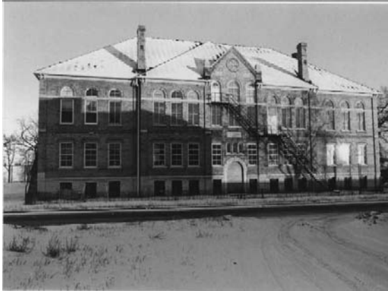
Original Northside Child Development Center, at Dupont and 14 th Avenue North, Minneapolis
