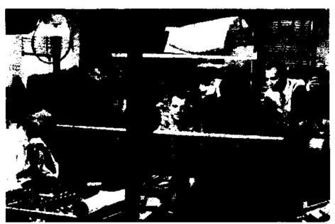
The group of individuals above are examining the MERLIN computer which was constructed at Brookhaven National Laboratory during 1957 to 1959. It was a high speed, general purpose, binary, digital computer modeled after the Los Alamos MANIAC II. The MERLIN was used by the Atomic Energy Commission in programs in the areas of chemistry, biology, and reactor studies. It was the first to be used as an on-line computer in a high energy physics experiment.
